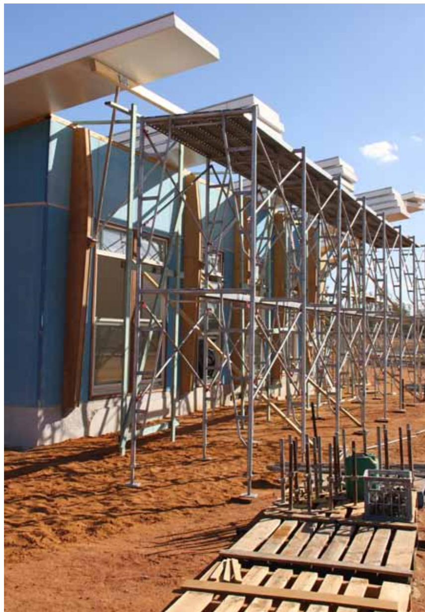
Perenjori flat pack housing pilot project
